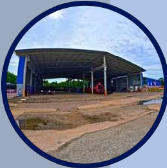
Workshop 2 Cranes 10 Ton Covered Operations 2,000 sqm
