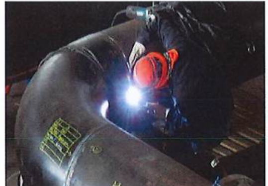
Pipe Spooling Welding
